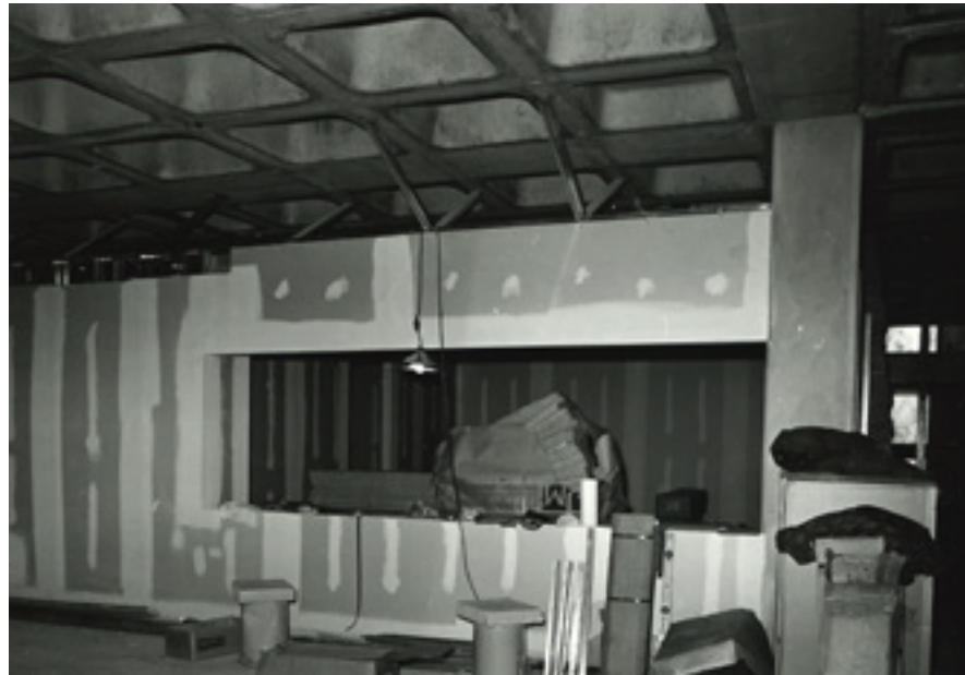
Construction of Dental Stores on the ground floor of the Dental Clinic Building, January 1978.
