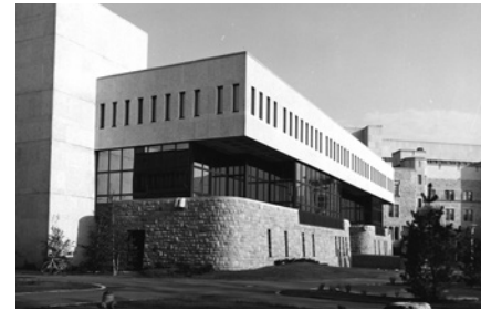
Exterior of the Dental Clinic Building in 1980.
